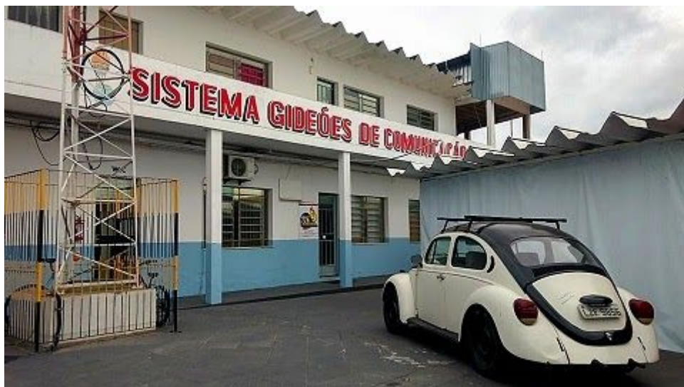
Photo: station entrance, the protection of the link tower can be seen.
