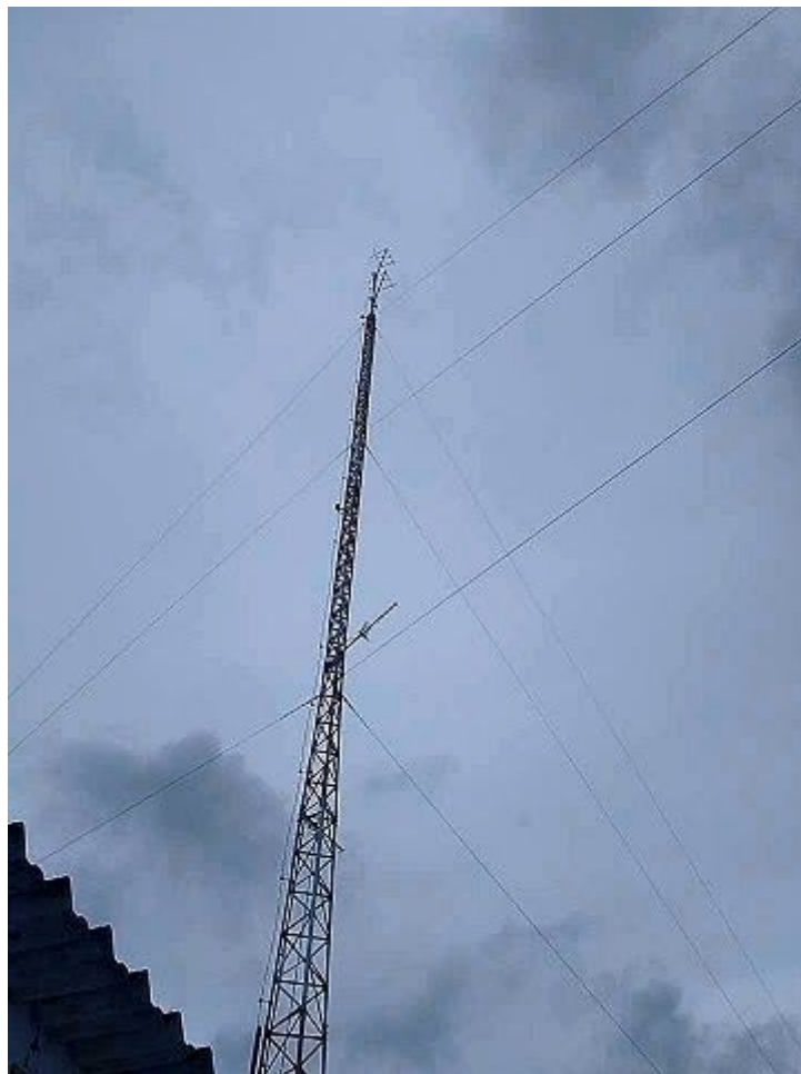
Photo: Radio links “Rádio Voz Missionária”, you can see at the top of the tower two dipoles of the Jampro type, belonging to the community radio station Rádio Paz no Vale 105.9 FM.
