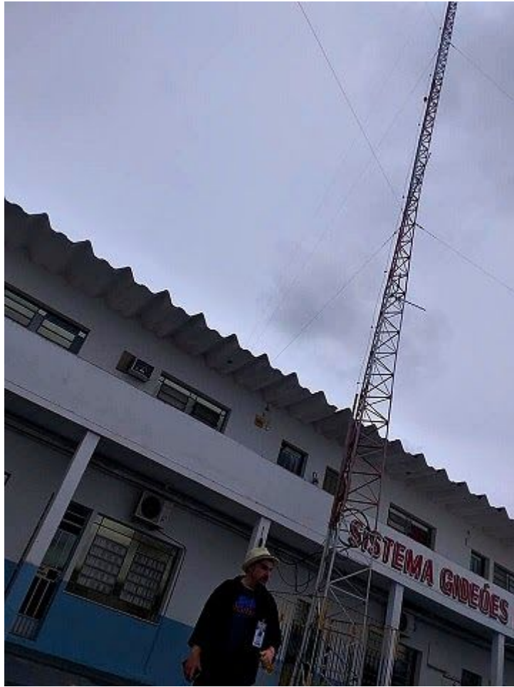
Photo: Martin Butera, next to the "Rádio Voz Missionária" link tower, you can see the Yagi antenna of the point-to-point system.
