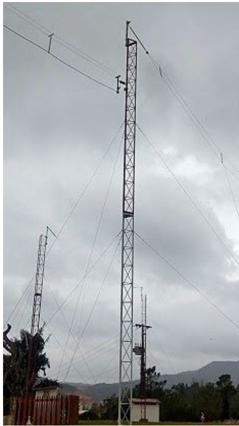
Photo: End of two Zeppelin antennas used by the broadcaster for different bands.
